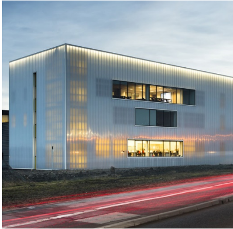
Polycarbonate façade panel - AMRC training centre
